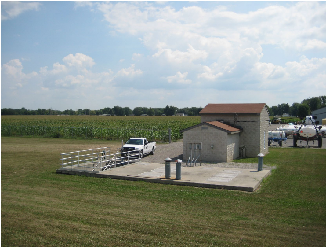
Franklin Street Storm Lagoon Pump Station with bar screen and wet well
